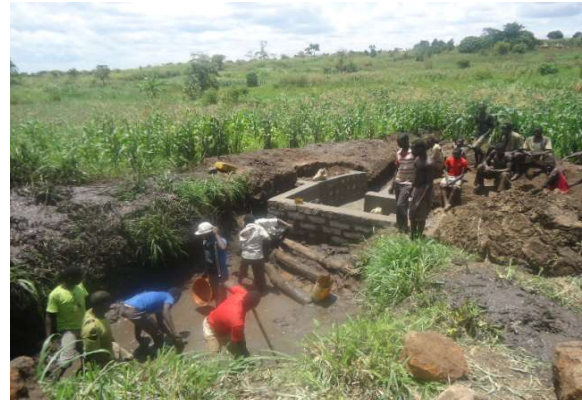
Spring well under construction
