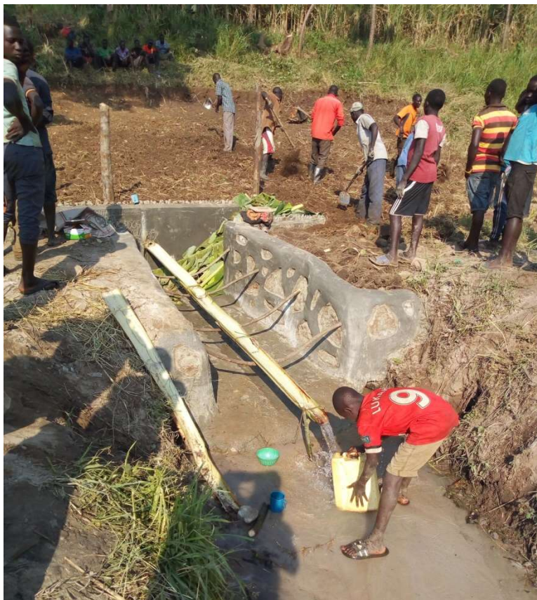
Edioivi spring well under construction, Masindi District, Uganda, January 2020
