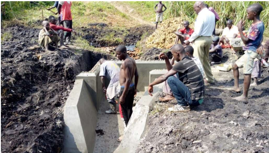
Constructing a clean water well, Masindi District, Uganda
